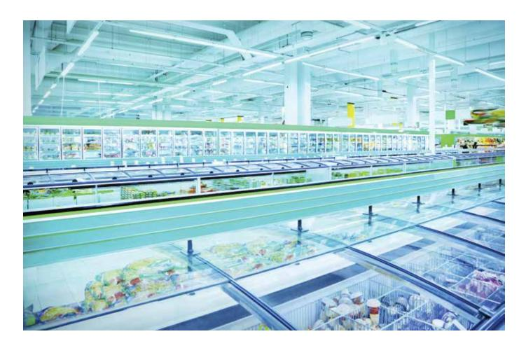
After the teams met, Raley's quickly identified an initial test store in Santa Rosa, CA for conversion to the newest low GWP refrigerant from Chemours, Opteon™ XP40 (R-449A). XP40 is a hydrofluoroolefin (HFO) blend that has zero ozone depletion potential (ODP) and a >65% reduction in GWP over the incumbent R-404A refrigerant. The team's project goals were to understand the retrofit details, validate operational performance, and measure energy performance of the new HFO refrigerant.
